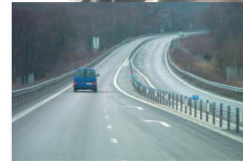
The provision of overtaking sections every 2km reduces driver frustration and the provision of a central safety barrier eliminates imprudent over taking. Provision for right turning movements will only be at designated junctions.
